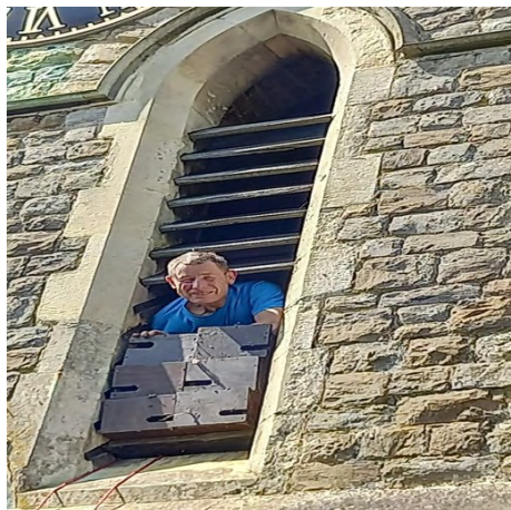
Six of the boxes being positioned in the tower
